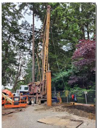
R-2 Well Drilling
